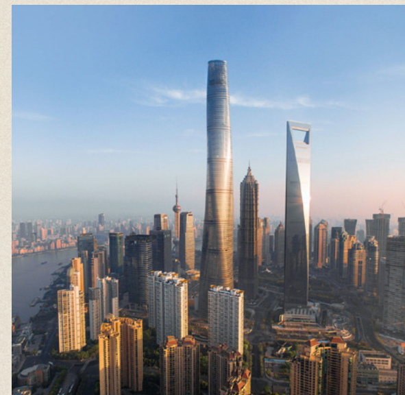
SHANGHAI TOWER, CHINA
