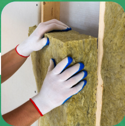
Insulation of Roof and External Walls
